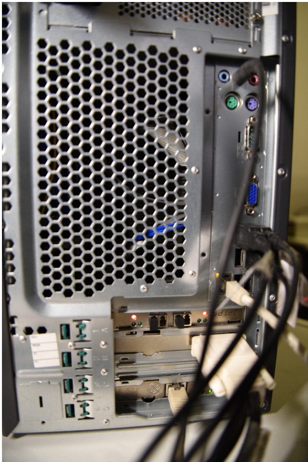
Figure 34: Example of a OPTPCI-e board horizontally installed in a Fujitsu Siemens Esprimo P7935. The board was de-installed in Oct 2020.
