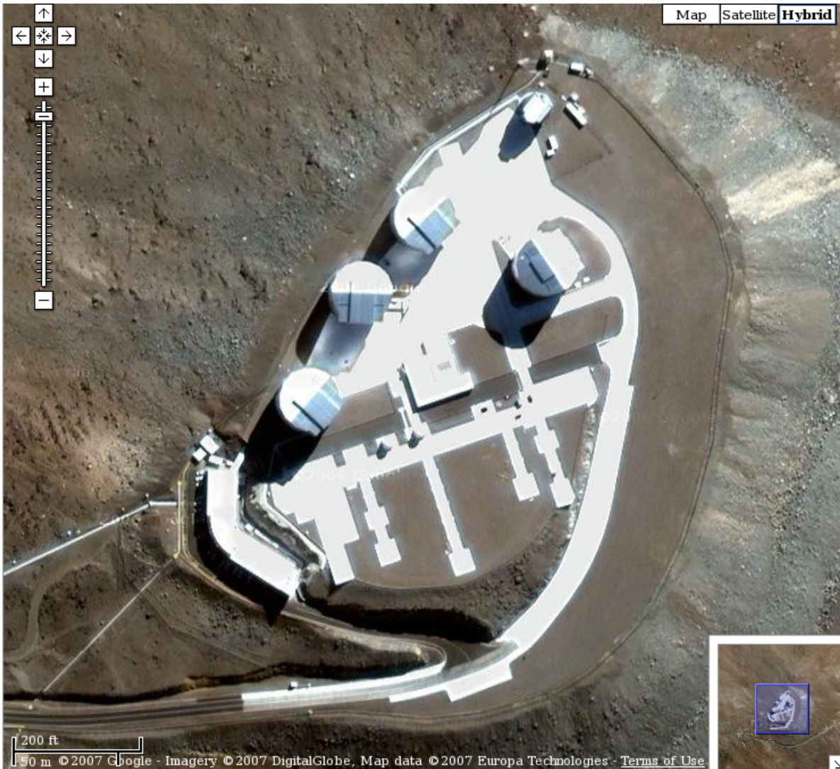
Figure 1: The picture indicates the location of the weather pole on the north rim of the platform by the long narrow shadow. In the NEVEC logo on the cover page, it is the red and white pin at the right. The VST dome is seen North of UT4.
